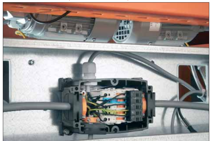
Centre infeed and distribution
