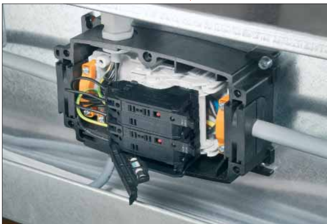
Circuit protection and distribution
